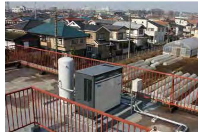
Component manufacturing plant: SMS11ED x 1
